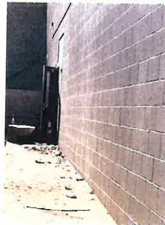
Photo 12 – Outside View Open Exit Door
