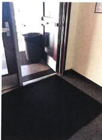
Photo 3 – Door Near 236 Hallway
