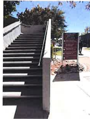
Photo 5 – SSV Exterior Stairs
